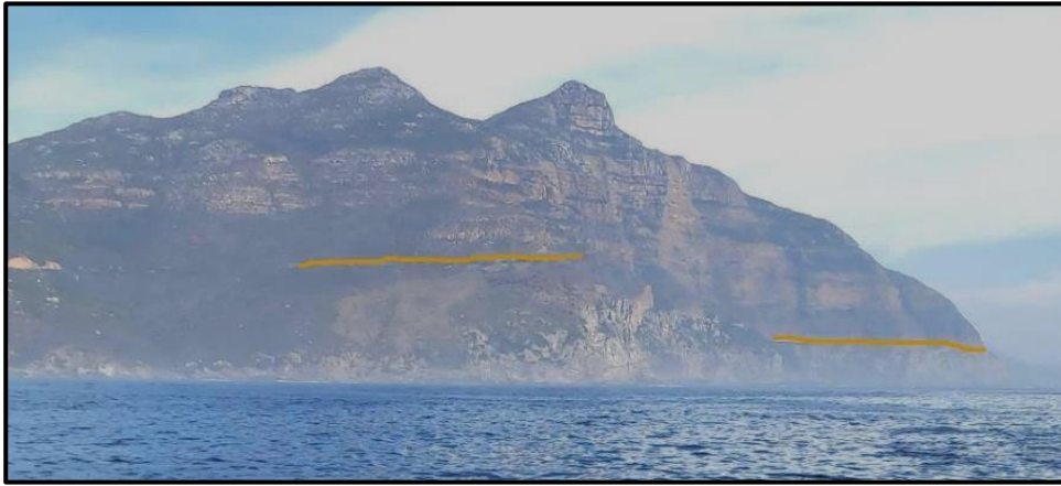
Figure 1: Chapman's Peak Drive Looking Southeast from the Sea
